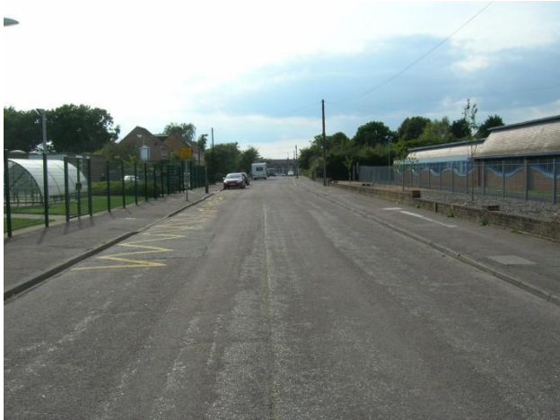
Plate 3.1: Footways on Hadow Road
